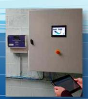
The control unit houses the pumping station protection, regulation and control instruments, as well as the frequency inverters to control the pump(s). The 2 air bubblers used for level control are also integrated in this unit.
